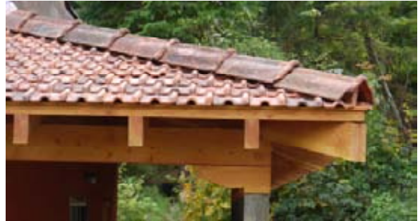
Vintage clay tiles, manufactured in France, were salvaged from Duncan's now-demolished Stonehaven and re-used in this hacienda-style portico for a ground-floor rental.
